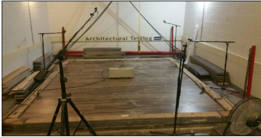
Source Room View of Test Specimen Installation
