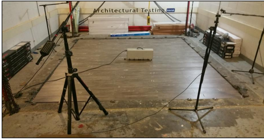
Source Room View of Test Specimen Installation
